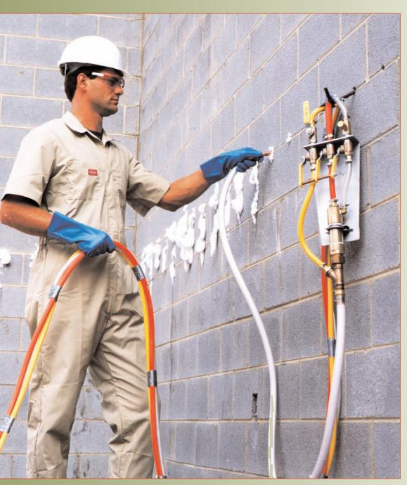
Core-Fill 500™ is a thermal and acoustical amino-plast masonry foam insulation with superior R-values, excellent sound absorption characteristics and enhanced fire-safety performance.
